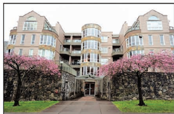
NOBLE HOUSE 2428 WEST 1ST AVE VANCOUVER, BC BUILT 1990
