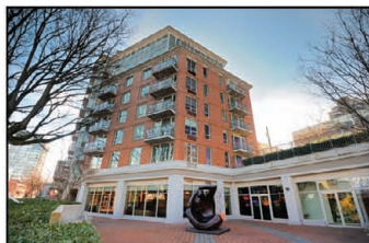
TERRACES ON 7TH WEST 7TH + FIR VANCOUVER, BC BUILT 1996
