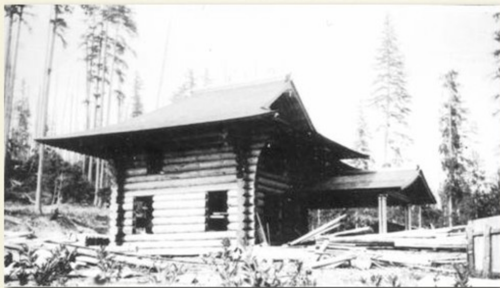
The "log cabin" under construction circa 1911
