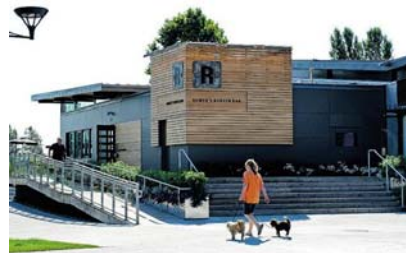
Serves as both a presentation centre and home to Romer's Burger Bar. Photograph by: Les Bazso, PNG, Vancouver Sun
