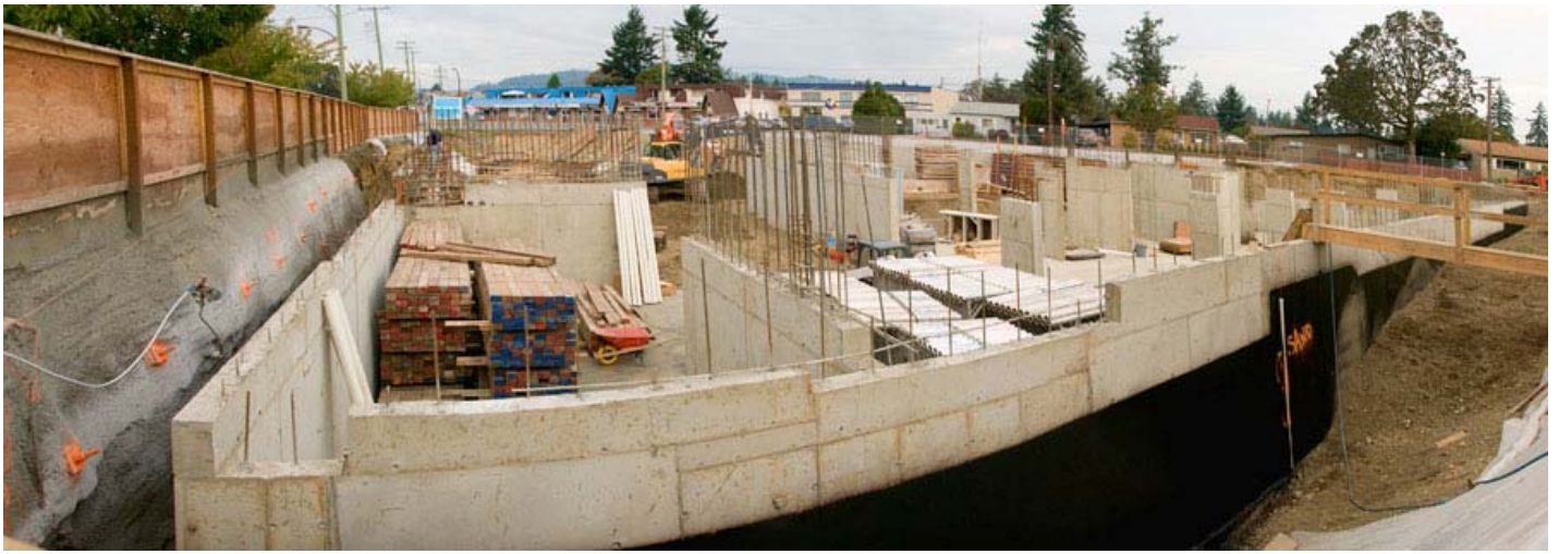
October 18th, 2010 - The foundation walls are nearly complete
