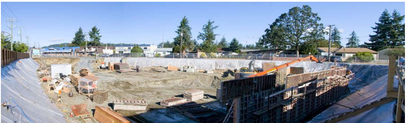
Construction view from Goldstream Avenue
