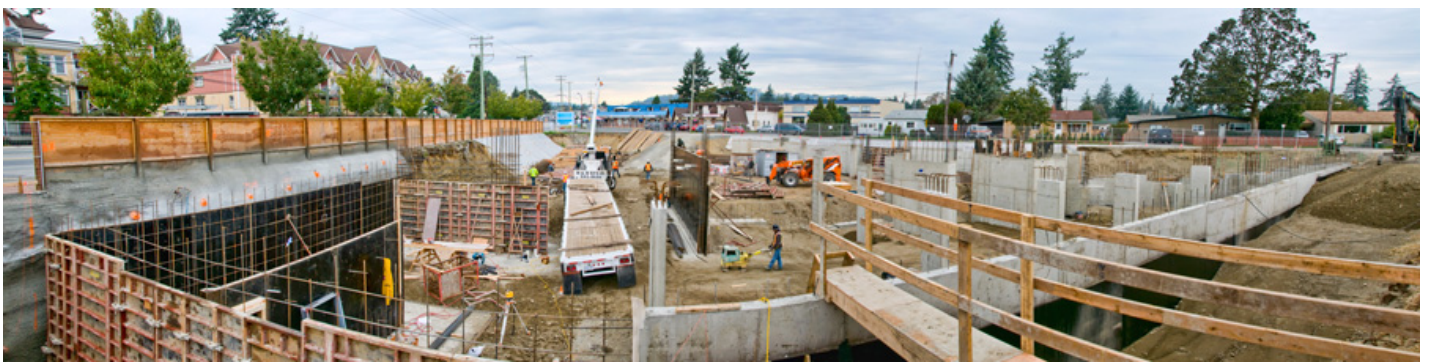
October 7th, 2010 - The foundation walls are going up
