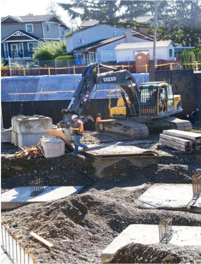
The first footings are in
