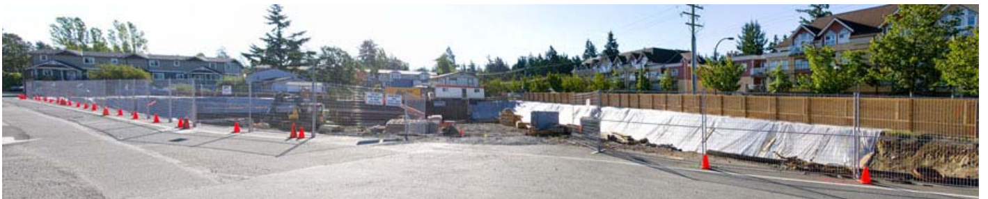
Excavation is complete. That's a big hole!
