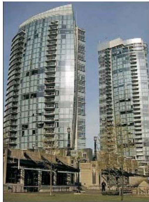
Carina/Callisto towers on West Cordova - glass towers
