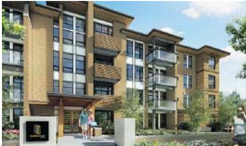
Glasshouse Lofts is a 67- suite, five- storey residential development built in New Westminster's Queensborough neighbourhood. The first occupants will move in in September.
