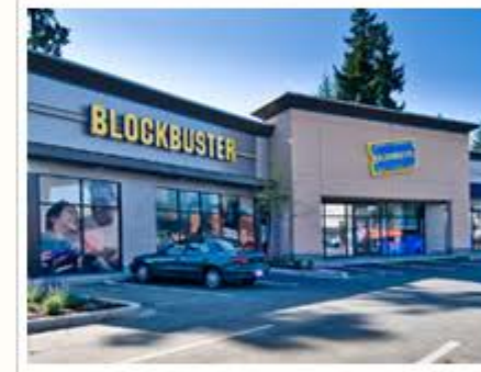
METRAL STATION Nanaimo
