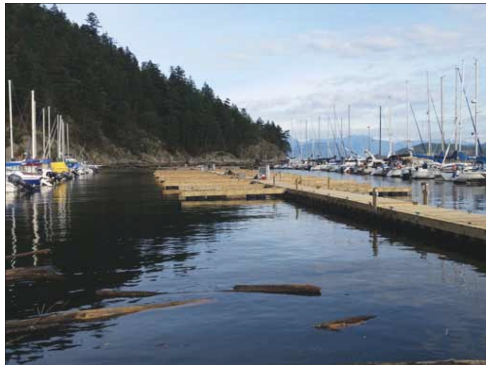
>>> Water crane at Sewell's Marina Spring 2014
