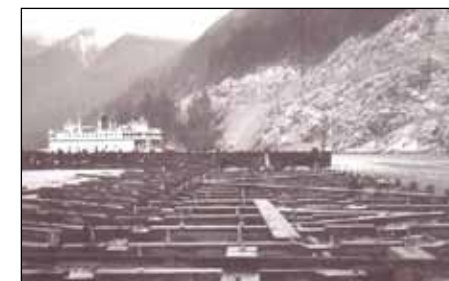
Installation of floating breakwater c. 1958
