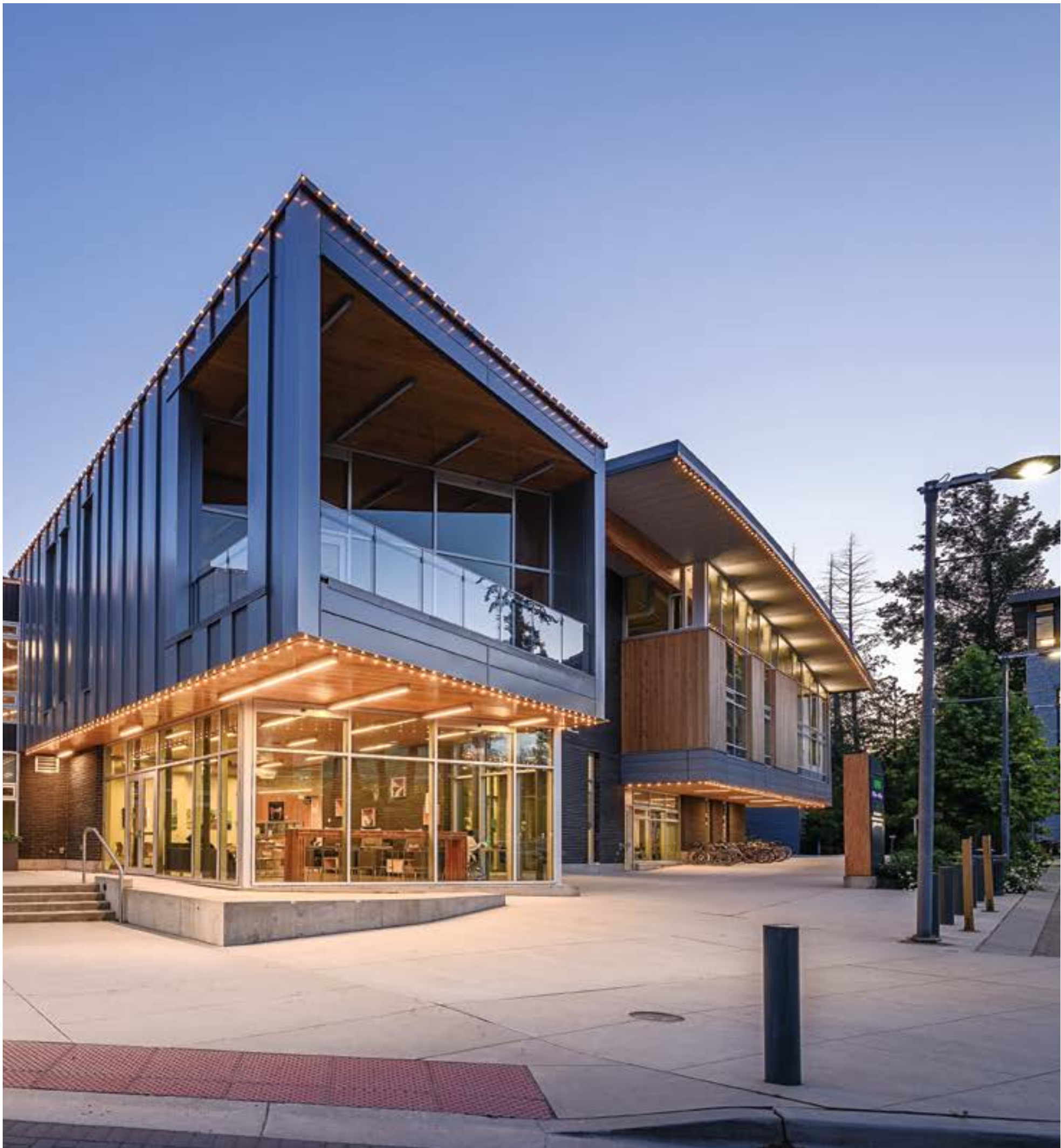
| WESBROOK COMMUNITY CENTRE |
