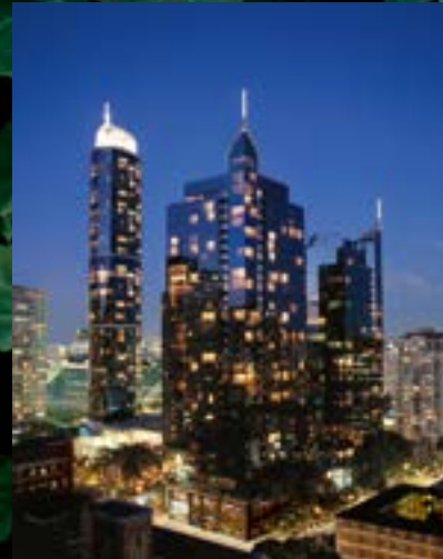
One Wall Centre | Downtown Vancouver
