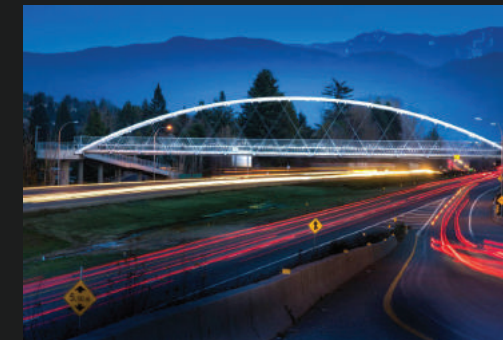
Salton Pedestrian bridge over HWY 1 3 min drive | 8 min walk away
